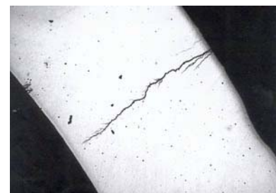
Figure 2. Cross-section of the crack
